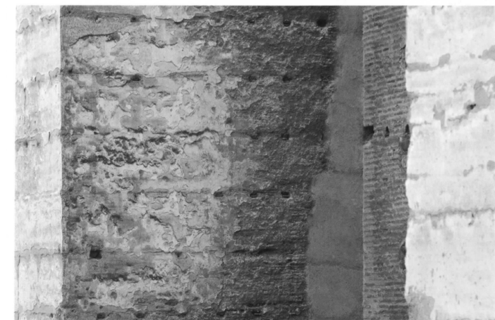
Figure 2 27 Nasrid rammed earth wall in the Alcazaba fort (Grabar)
